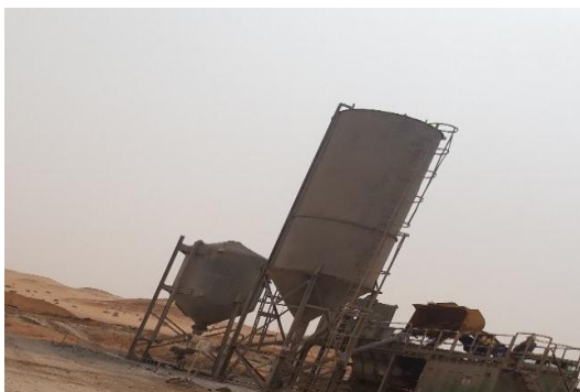
Figure 23 : silo de ciment
